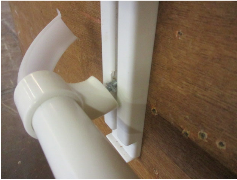
Photo 7: KiddieRail. Test 3 – Point Load. At 25Kg, bracket detached from wall mount.
